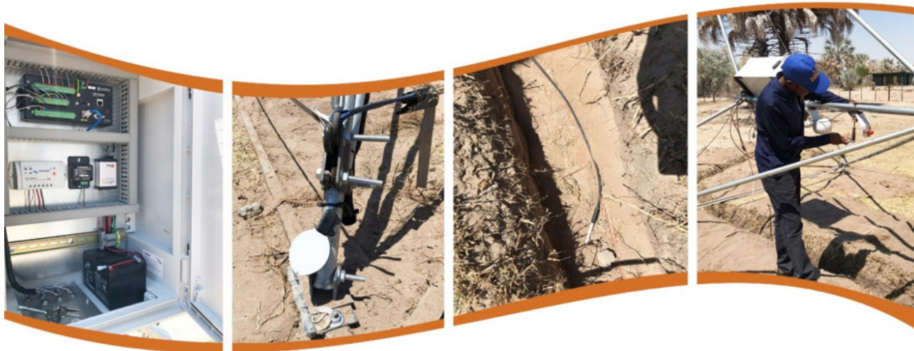
Installation of new Automatic Weather Station in Omafo in the Ohangwena region, Namibia
